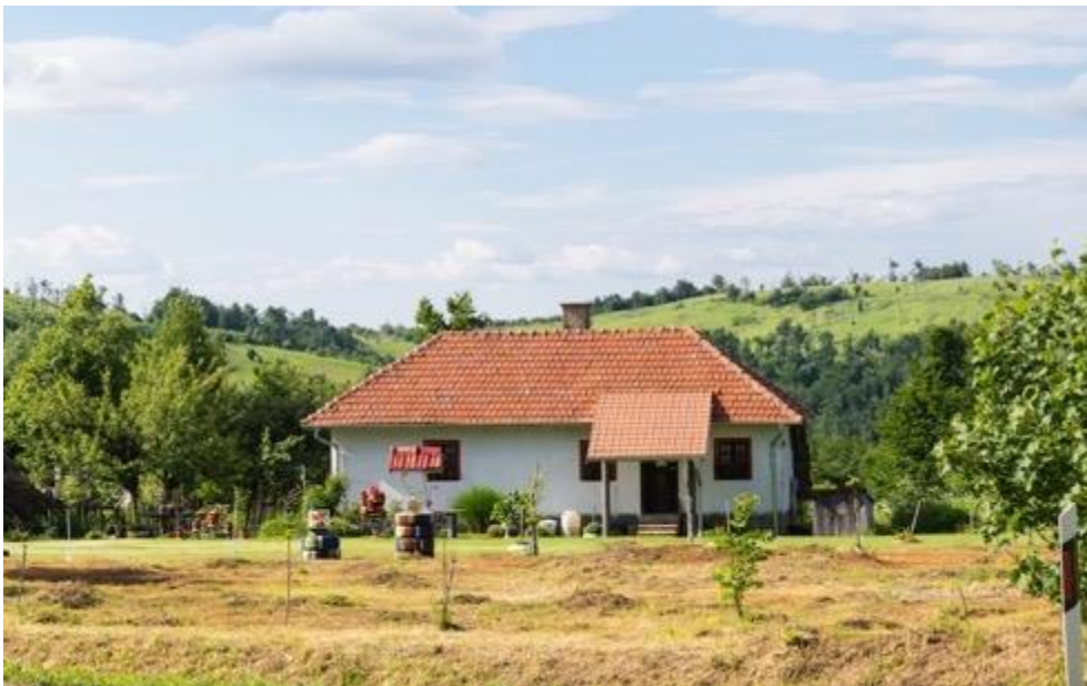
Figure 14-3 Weekend House in the Central Part of the WPP Site
