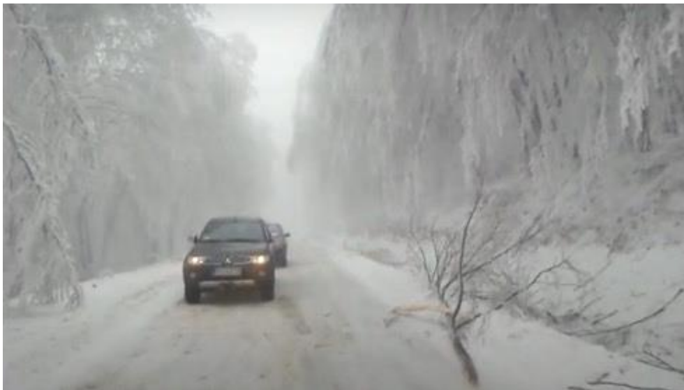
Figure 14-18 Winter Driving Conditions on the Public Road No. 161 in Crni Vrh 60
