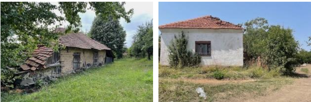
Figure 14-6 Dilapidated Structures in the Study Area
