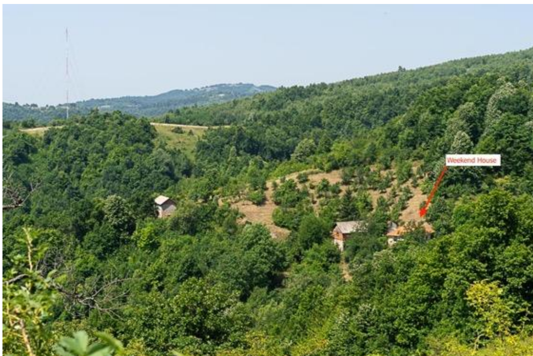
Figure 14-11 Weekend House W1 West to the K3 Met Mast and Proposed Turbine TIV-1
