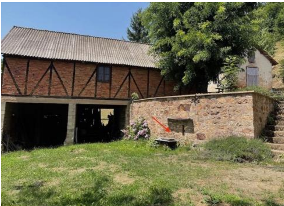
Figure 8-10 Tapped Low-Yield Groundwater Source East of the Site
