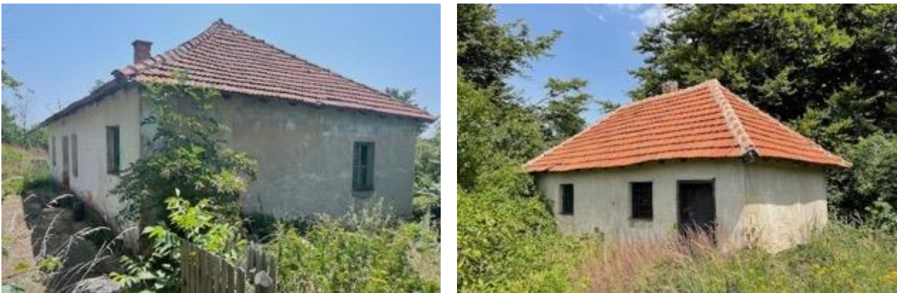
Figure 14-5 Abandoned Houses in the Study Area
