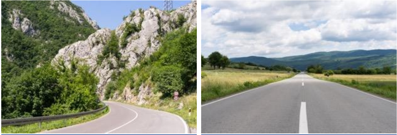
Figure 8-80 Public Road in the Gornjak Gorge (left) and in Žagubica Valley (right)
