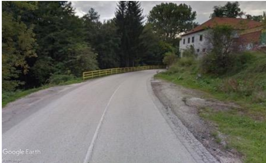
Figure 13-2 Typical Blind Bend on the Road No. 161
