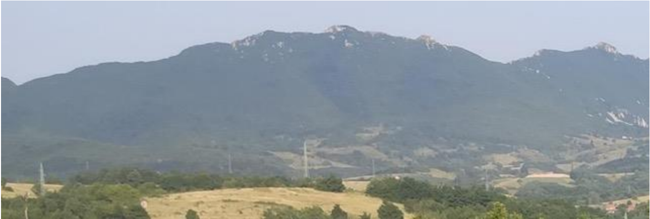
Figure 8-29 Veliki Krš Mountain – View from the WPP Site Eastern Boundary
