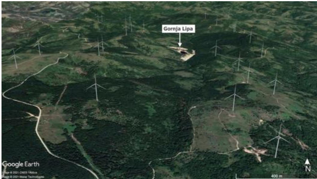
Figure 8-12 Perspective View of the Proposed WPP and Gornja Lipa Abandoned Open Cast Pit
